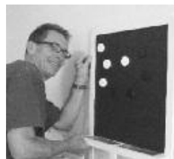
Rebuilding Together Construction Captain, Ken Rhoads, hangs up a chalkboard in the playroom. Ken did extensive work to prepare for the big makeover day, including building a desk for the new study room.
